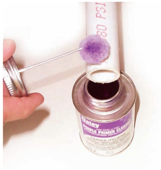
FIGURE 18-35 Apply PVC cleaner. Courtesy of Larry Jeffus.
