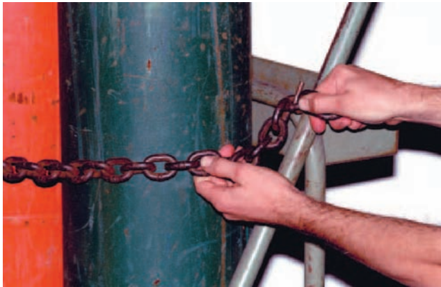
FIGURE 3-45 Safety-chain the cylinder. Courtesy of Larry Jeffus.
