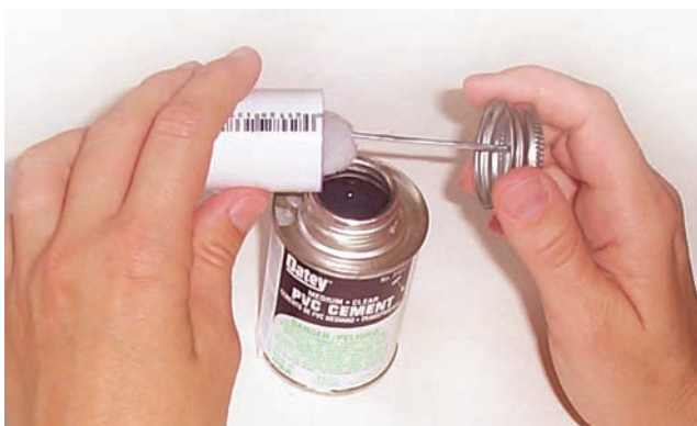
FIGURE 18-77 Apply PVC solvent to the inside of the coupling. Courtesy of Larry Jeffus.
