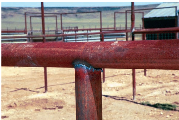
FIGURE 10-51 Pipe joint cut and fitted, ready for cleanup and welding. Photo courtesy of Larry Jeffus.
