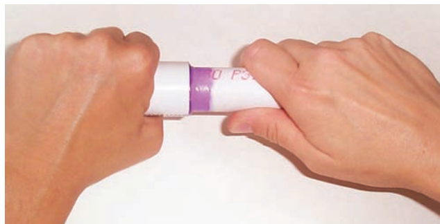
FIGURE 18-78 Insert the pipe into the fitting; then rotate 90 degrees and hold for 15 seconds. Courtesy of Larry Jeffus.
